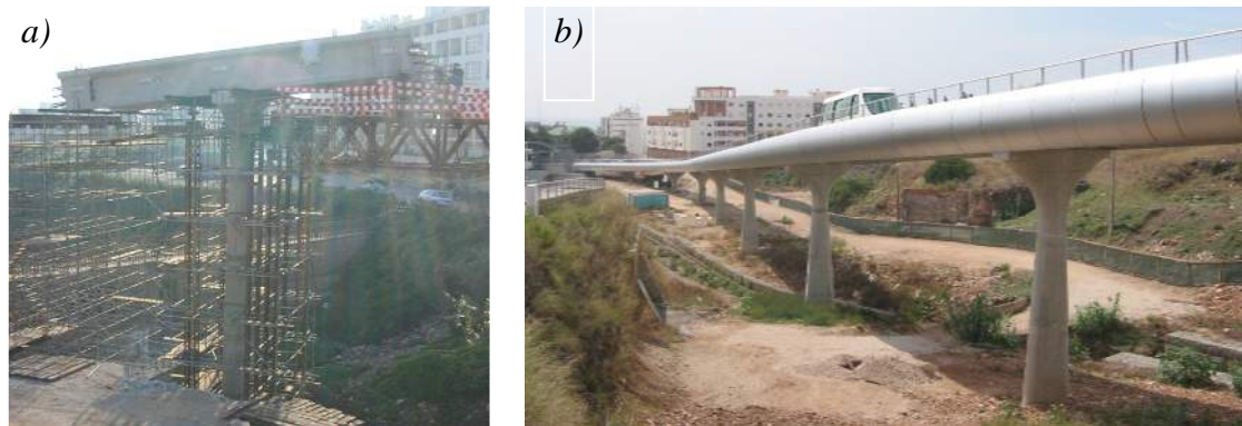
Fig. 4 – Construction phase and final view of the first viaduct in service
