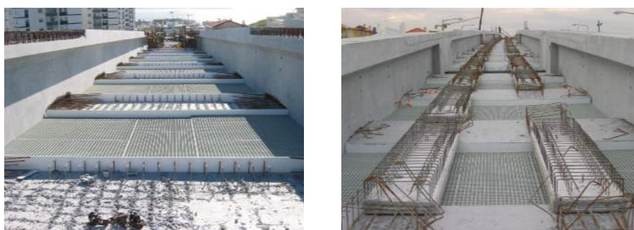
Fig. 3 – Construction phase of the connections between the prefabricated elements
