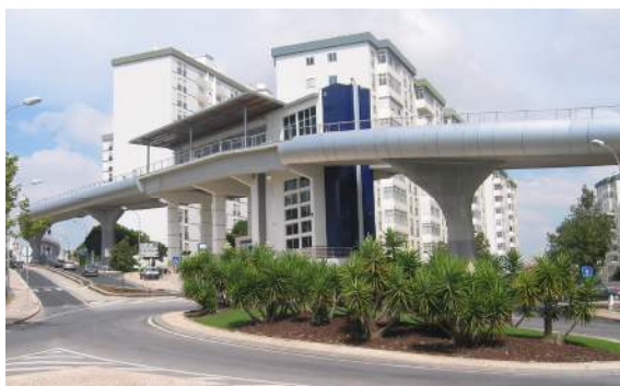
c – Middle station and connecting viaducts
