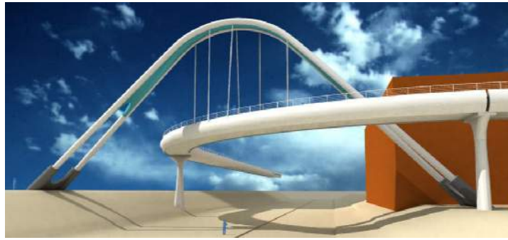
Fig. 6 – Preview of the start of the third viaduct with the metallic arch
